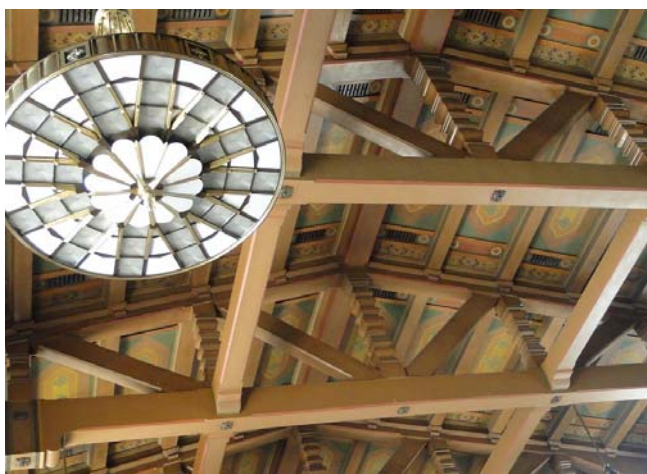
Ceiling and chandelier in the old ticketing area
