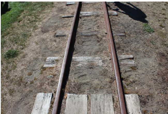
An example of "low cost" 2' trackage
