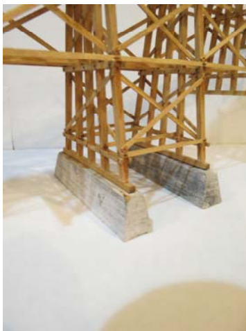
Completed foundation under the tall bents of the bridge
